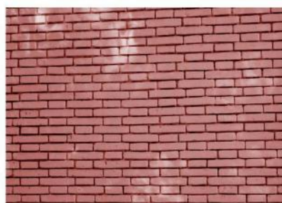
(a) Brick wall
